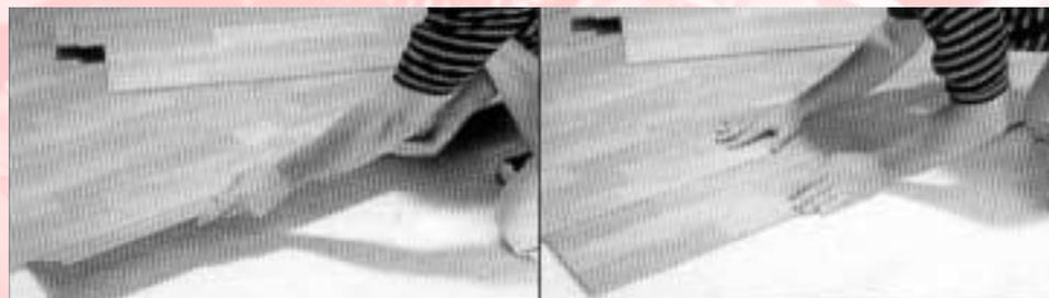
UltraLock: A patented form of tongue and groove firmly locks the elements together, both lengthwise and crosswise. It is faster and easier to lay the floor whether it is done by a professional or a do-it-yourselfer.
